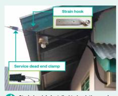
Strain hook is installed to hook the service dead end clamp. The type of strain hook depends on the surface material.
