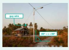
Pole is installed firmly and stabilised with guy wire.
