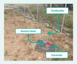
Guy-wires are anchored securely using turnbuckle hooked on the anchor head. Turnbuckle is used to adjust the tension.
