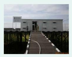
Power house and PV array are installed on top of the wooden patform to avoid disturbance caused by water.
