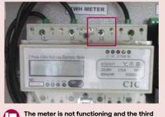
line is not connected to the meter. Fuse might be blown.
