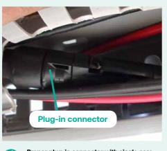
Proper plug-in connector with single core cable is used. Cables including the connectors are also located inside cable tray.
