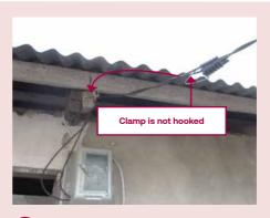
Incorrect use of service dead end clamp. The clamp should be hooked on the strain hook.
