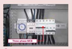
Three-phase MCB is used for three different feeders. Fault in one feeder will unecessarily disconnect all feeders.
