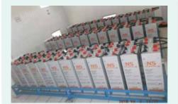
Strong battery rack with no sign of corrosion. Rack is equipped with side bar to protect battery from falling
