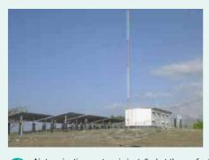
Air termination system is installed at the perfect location to cover the PV arrays and power house.
