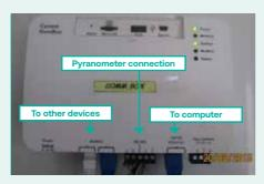
Functioning monitoring system with connection to the other devices through Xanbus and RS485 for pyranometer.
