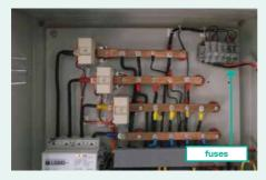
Voltage measurements are protected by fuses.
