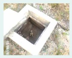
Grounding electrode is installed in moist soil. Higher moisture content may increase significantly the soil conductivity.
