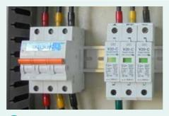
Neat installation and proper cable shoes are used.
