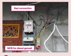
Poor and dangerous installation. Cable connection shall comply to local standard and fixed to the wall .
