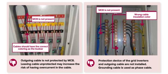
Every grid inverters and outgoing cables must not be left unprotected. Proper type and size of protection device is crucial in providing safety in the installation.
