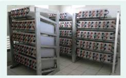
Horizontal battery arrangement on hot deepgalvanized steel rack structure with no sign of corrosion.
