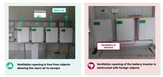
Ventilation opening of the battery inverter should never be blocked by any object to avoid unnecessary increase of heat. Increasing of heat will reduce the output power. Battery inverter ventilation openings must regularly be cleaned from dust deposits
