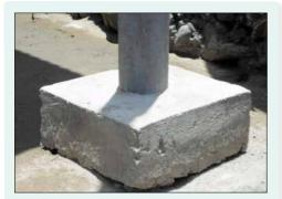
The concrete foundation is not burried but is placed on a flat surface of other solid concrete foundation. However, a ballast foundation is acceptable only and only if it fulfills some preconditions<sup>10</sup>.
