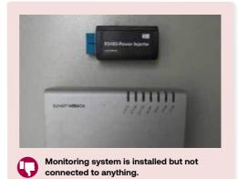
Ensure that all the monitored devices are connected to the bus. There is a maximum number of connected devices on a single monitoring device that should be taken into account. Consider having additional monitoring device and creating multi-cluster configuration when maximum number is exceeded.
