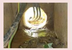
Puddle and dirt inside the tunnel due to unsealed cable tunnel. The uncovered tunnel may become the entrance gate of rodents and reptiles.
