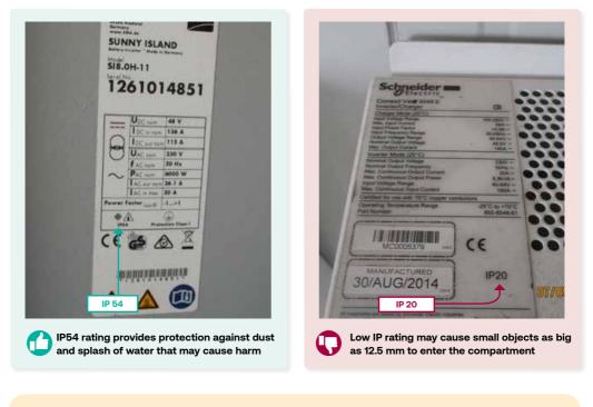
The information on the label is useful to identify the type and electrical characteristics of the installed battery inverters, especially during inspection or maintenance. Label should be attached and easily visible.
