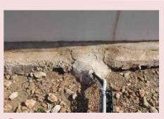
Cables are installed on the ground without any protection from sun exposure. Cement is used to seal the cable entry.
