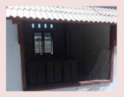
Poor ventilation opening. Smaller net should be used instead. Grill should be provided to ensure the security.
