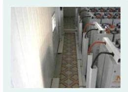
Cables are installed neatly inside cable conduit. Correction factor of enclosed and grouping installation should be applied according to IEC 60364-5-52.
