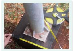
Very good quality foundation with plastered concrete, perfect dimension, and firmly fixed to the base plate by the anchor bolts.
