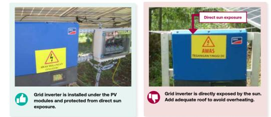
To avoid overheating components, grid inverter must be protected from direct sun exposure. Increasing temperature may reduce its performance and life expectancy.
