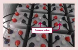
Broken battery valves will expel some the gasses easily to the atmosphere and reduces capacity of the battery
