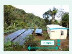
Separation distance is kept between the down conductor and PV modules frame and power house.
