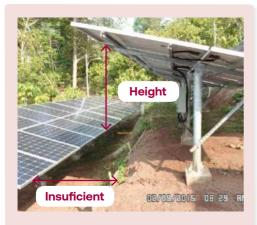
Insufficient distance between arrays leads to partial shading on the lower array.
