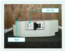
An 1 Ampere MCB is used to protect household installation. This equal to roughly 230 W of power consumption.
