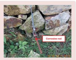
Poor installation of the grounding rod inside pile of stones. The unburied rod does not provide any intimate contact with earth.
