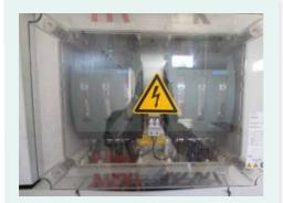
Enclosure is made from polycarbonate that provides good insulation and properly labeled with electrical shock hazard.
