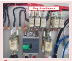
Very close distance between positive and negative busbar. Rearrangement of components is required.
