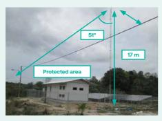
PV arrays and power house are inside the protected cone of the air termination system.
