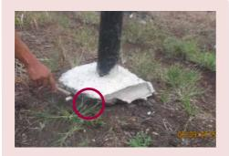
Gap between concrete foundation and the ground. Concrete foundation is constructed without any functional use.
