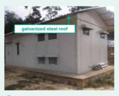
Power house made of lightweight prepainted galvanized steel with polyurethane foam as insulation material.
