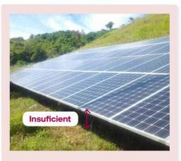
PV array is too low. Vegetations may shade the PV modules and reduce the airflow below the module.
