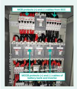
Battery banks, SCCs, and battery inverters are protected by MCB and MCCB on both positive and negative sides.
