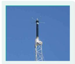
Early streamer emmision (ESE) rod is used to enlarge the protection radius and improve the precision using additional ionization system.
