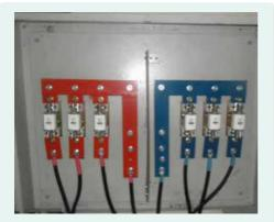
Adequate distance between the busbars. Separator is provided to avoid accidental short circuit during installation or maintenance.
