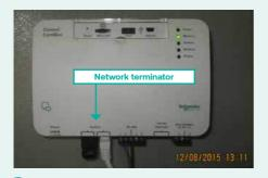
Network terminator is installed to the remote monitoring, the component is the first component of the system that connects to the network
