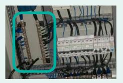
Adequate distance between line and neutral busbars.
