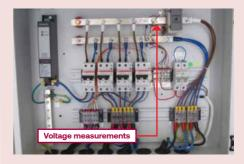
Voltage measurement is not protected by any protection device. Energy meter is not installed.
