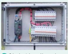
Polycarbonate box provides a good insulation in case of electrical fault. Additional grounding is not needed.
