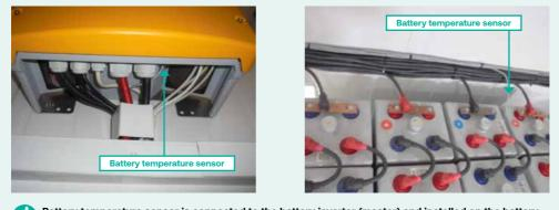
Battery temperature sensor is connected to the battery inverter (master) and installed on the battery for charging compensation feature.
