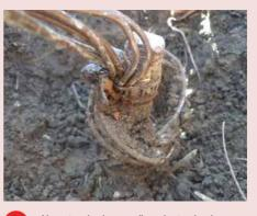
Non standard grounding electrode clamp is used. Corrosion may not only cause resistance to increase but also break the connection
