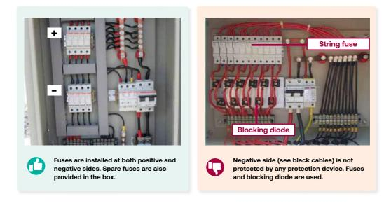
Opt to use a string fuse instead of blocking diodes. Blocking diodes cause additional drop of voltage for about 0.5 to 1 V that leads to significant power losses. The function is better served by a string fuse.
