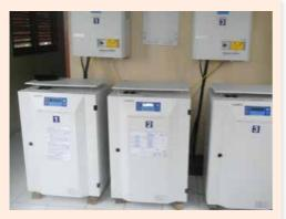
One SCC is not installed. Missing SCC will reduce the energy production from the PV thus limiting the energy supply to the load.
