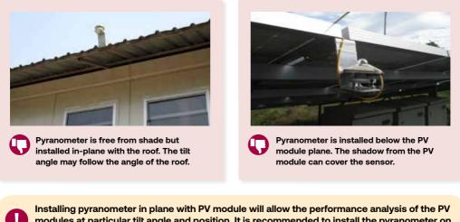
modules at particular tilt angle and position. It is recommended to install the pyranometer on top of the PV array structure to avoid shading of the PV module from any angles.
