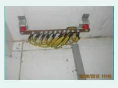
Equipotential bonding bar is installed properly with secure connection of grouding conductors.
