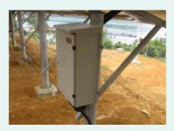
Combiner box is located under the PV module to avoid direct exposure from sun and rain.
