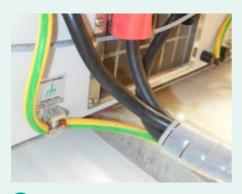
Grounding connection of the exposed conductive case is provided to prevent electric shock.
