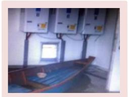
Flooding in power house may cause electrical faults, damaging the electrical components and endanger the operator due to electric shock.
