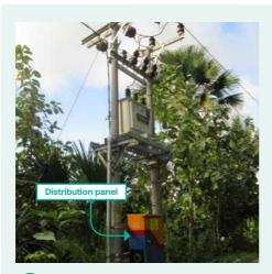
Panel distribution is installed to distribute power to feeders and protect low-voltage side of the transformer.
