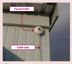
The pyranometer has probablity of being shaded and thus providing unreliable global irradiance data.
