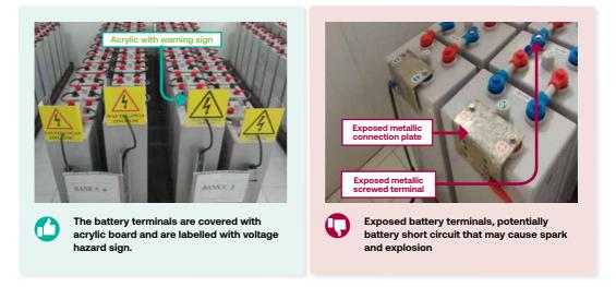
The terminals of the battery are always alive, therefore never leave the terminals unprotected. Metal parts may cause accidental short circuit. It is recommended to use insulated wrench when fixing the connection.
