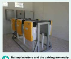
Battery inverters and the cabling are neatly installed and routed inside the cable conduit.
