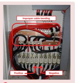
Preferable installation with horizontal busbar arrangement. It provides easier cable routing and clear separation. Vertical busbar arrangement makes difficulty to arrange and route the cable. Some positive cables touch negative busbar and vice versa.
