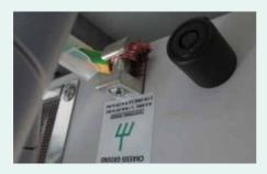
Chassis of the battery inverter is grounded through lay-in grounding lugs.
