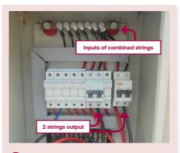
Strings are combined in the combiner box and split equally to be used as input of grid inverter.
