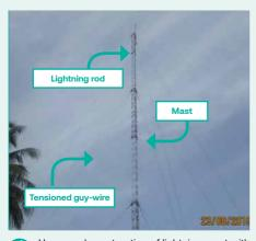
Very good construction of lightning mast with guy-wire to add stability on the free-standing segmented mast.
