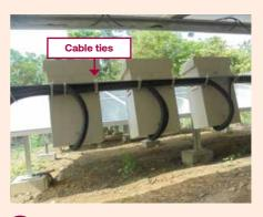
Unstable and poor installation, the cable ties may not be able to hold the load.
