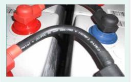
NYAF 50 mm<sup>2</sup> cable is used to handle maximum of 104 A. A correction factor due to ambient and grouping used is 0.75.
