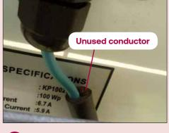
Make-shift solution of using only single wire from multi-core cable.
