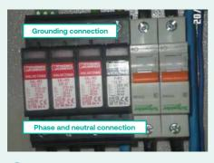
Phase, neutral, and grounding cables are properly connected to the surge protection device.
