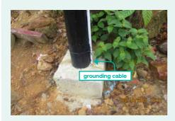
Pole and neutral conductor are grounded with sufficient grounding cable to maintain the TN-C configuration.
