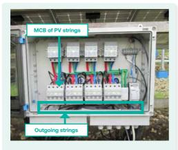
Strings are individually go to the grid inverter. MCB serves as overcurrent protection as well as diconnector.
