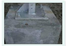
Base plate is used at the bottom of the pole to anchor the pole to the foundation and increase stability.
