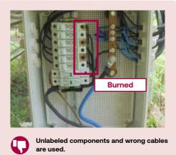
Difficulties in conducting service or troubleshooting are often found when tracing and finding the correct components. It is recommended to label all components and put the circuit diagram at the door of combiner box.
