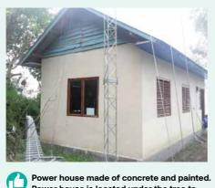
Power house made of concrete and painted. Power house is located under the tree to shade from direct sunshine and keeping the temperature low.
