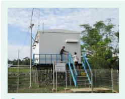
Power house is installed at higher level to avoid water from entering the power house during flooding.
