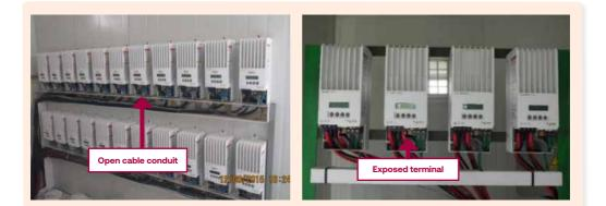
Exposed terminal of solar charge controllers. High voltage DC may exist at the terminals and cause an electric shock. The network power cable should not be routed together to avoid noise in the communication.
