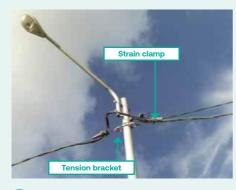
Strain clamps are used to hold the overhead cables. Certain length of cable should be remained to adjust the cable tension.
