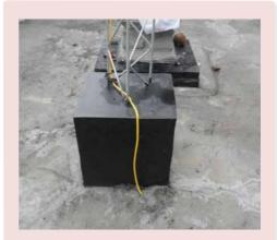
Grounding electrode should not be installed directly in the concrete. As its temperature may rise and cause concrete to break.
