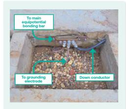
Equipotential bonding bar to connect between lightning grounding electrode and main grounding system.
