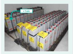
Battery cells are installed with sufficient distance for the battery to release heat.
