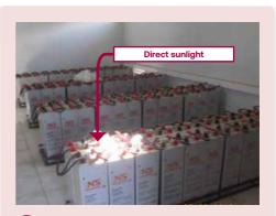
Some batteries are exposed directly to the sun light. Long term heating may cause those specific batteries to fail earlier.
