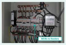
Single phase MCB is used to protect individual feeder.
