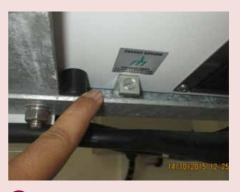
Chassis of the battery inverter is not grounded. Ungrounded metal case may lead to electric shock hazard.
