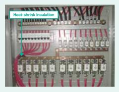
Adequate distance between the component and bigger internal space allows the electrical components to dissipate heat.
