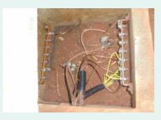
Good installation of grounding electrodes and equipotential bonding bar with adequate distance from the ground.
