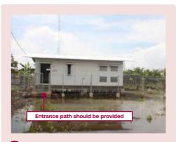
PV mini-grid installed on muddy and watery land with inadequate pathway to access power house and PV array.
