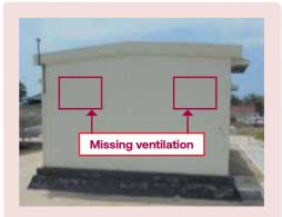
Insufficient ventilation to provide air circulation inside the battery room and to keep the room temperature low.
