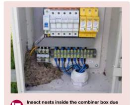
to poor ingress protection (IP).
