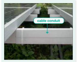
Cables are protected inside the cable conduit. Providing cable support may increase the lifetime of the cable.
