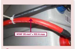
Undersized NYAF cable is used in the battery string that could be charged with higher current than the cable rating.
