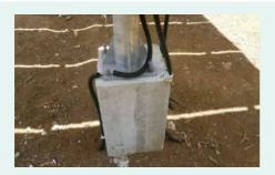
Mounting structure is bonded to the PV module frame and neatly grounded.
