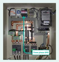
Three phase surge protection device is installed in the panel to protect the installation against overvoltage
