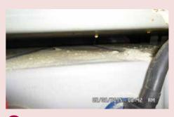
Sulphide flakes may cause corrosion to battery rack. Clean the battery and reduce the charging voltage if necessary.
