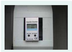
Battery powered lightning counter is in operation and protected from harsh environment inside the box.
