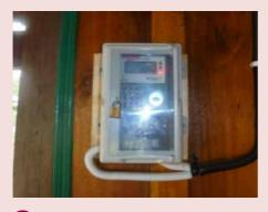
For security and safety reason box should be locked and only operator has access to the box. However, MCB should not be installed inside the box.
