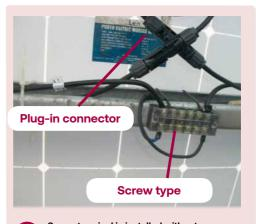
Screw terminal is installed without any protection. Exposed terminals lead to serious electric shock hazard as well as electric faults.
