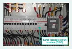
Correct installation of the ELCB. All the phases and neutral are connected to the ELCB.
