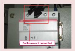
Cables are not connected to the surge protection device. The system may not be protected from voltage spike.
