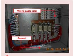
Ungrounded box and improper way to seal the cable insertion. Use of sealant will make cable installation become semi-permanent. How to improve the quality of the panel?
