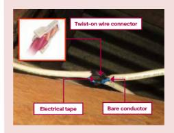
Junction connection is not installed inside box. Twist-on wire connectors should be used to fasten the conductors instead of electrical tape.
