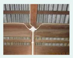
Neat cable installation and junction. NYM cable and conduit is used for household appliances.
