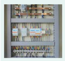
Cables are neatly wired and routed inside cable tray. Colour codes and labels are used to identify phases and components.
