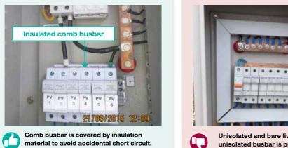
Unisolated and bare live conductor or unisolated busbar is prone to have short circuit.
