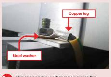
Corrosion on the washer may increase the connection resistance. Avoid direct contact of dissimilar metal that has different anodic potential.
