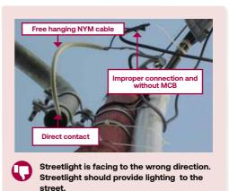
MCB must be installed to only disconnect individual streetlight in case of short circuit due to faulty device. A combined type 1 and 2 surge protection devices must also be installed on the streetlight pole that has grounding installation.
