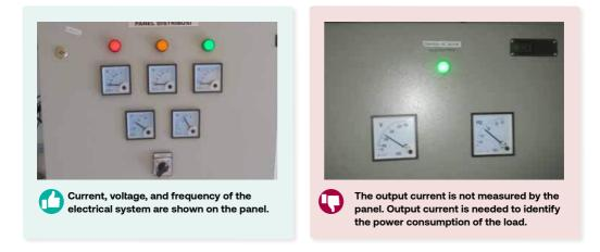
Voltage and current measurement of the output should at least be installed on the panel to display the power delivered to the loads. The information is useful for the operator or technician to see the instantaneous power as well as to detect faults.
