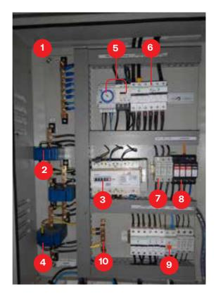
30 kW AC distribution panel with three-phase configuration
