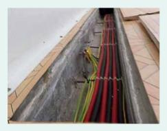
Grounding and cables are installed neatly with direct laying method.
