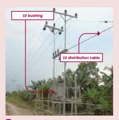
LV distribution cable is not protected by any protection device. Cables from LV bushing is directly connected to the LV distribution line.
