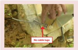
Makeshift solution using nails to fix the earthing electrode on the mounting structure
