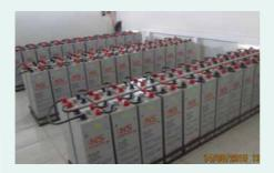
Battery are installed inside th battery rack with edges to avoid the battery from faling.
