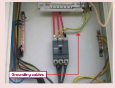
Wrong insulation colour (grounding cable) is used for the line phase. Correct colour should be used instead.
