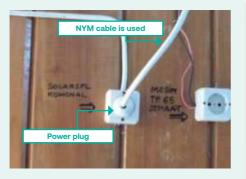
AC power plug with correct cable type is used. Grounding terminal and cable must be connected when the device requires grounding.
