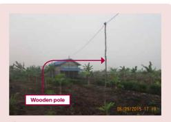
Low-voltage distribution cable is hanged on the thin wooden pole due to the extended distance between metal poles.
