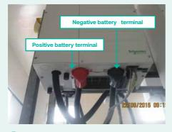
Battery terminal connection is protected with insulator material from direct touch and being shorted.
