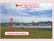
Massive installation of lightning rods may cause additonal shading on the PV modules.
