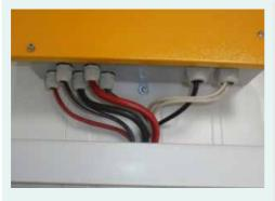
Cable glands are used to protect the cable and prevent animal entering the compartment.
