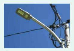
Waterproof LED streetlight with IP 65 rating is used.
