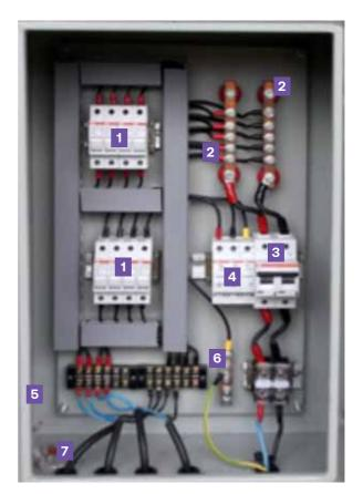
All components in the combiner box is operating in DC voltage that may reach up to 1,000 VDC, depending on the grid configuration. An AC-coupling system with grid inverter typically has higher input voltage of up to 1,000 VDC, while a DC-coupling system with solar charge controller is in the range of maximum 150 VDC. It is preferable and safer to have a lower voltage in PV mini-grid, although higher voltage system will reduce the losses in the circuit.
