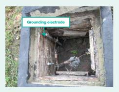
Grounding electrodes are connected in parallel to reduce the grounding resistance. However, the distance should not be too close
