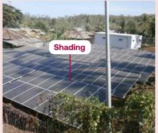
Shading from big trees around could significantly reduce the power production up to 40%.
