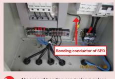
Absence of bonding conductor may lose the protection against indirect contact as well as protection from lightning strike
