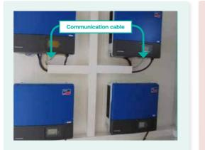
The communication of grid inverters are interconnected through RS485 in daisy chain configuration or in series
