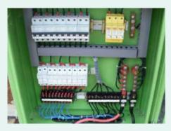
Proper dimension of combiner box. The bigger internal space allows the electrical components to dissipate heat.
