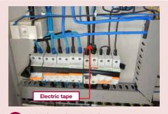
Cable is not installed with proper cable shoes. Eletrical tape is used as insulation and to fix the MCBs.
