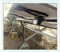
Neat wiring with fixed installation of connection box. Quality of the internal connection must be verified during inspection.
