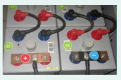
Battery terminal is in good condition and is free from corrosion or sulphate flakes
