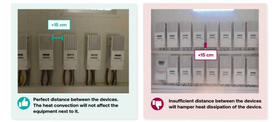
Sufficient distance between the SCCs should be provided to allow heat to dissipate. Rated performance may not be achieved if the clearances are below the requirement.
