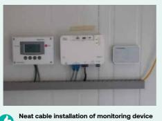
Neat cable installation of monitoring device and system control panel. Router will only be used when remote monitoring via GSM/ GPRS is possible.
