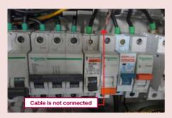
Improper connection may lead to an electric arc. MCBs are not equipped with labels.
