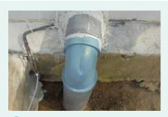
Cables from combiner box are installed undergrond and protected inside PVC pipe.
