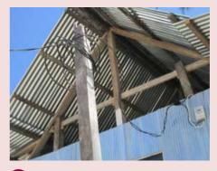
Unnecessary long cable to the household without any proper cable support. The longer the cable, the higher the losses.
