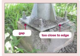
Undersized foundation may not be able to withstand high mechanical load and possibly the reason of the cracks.
