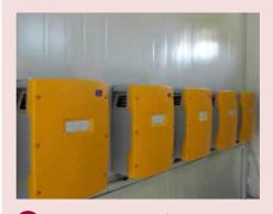
Absence of label on the inverters can cause difficulties when carrying out inspection or maintenance
