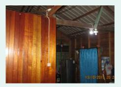
Lamp fixture is mounted on the beam and switch are installed at reachable height. Cables are well mounted on the wall and without tension.
