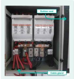
Cable gland is used to prevent animal enrtering the panel.
