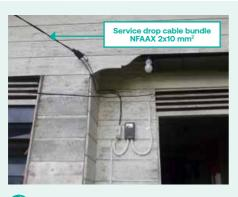
Service drop cable is under tension and cable is well installed on the wall using cable clamp.
