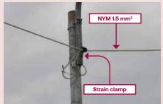
NYM cable is used as overhead distribution line. Cable with crosssectional area of 1.5 mm<sup>2</sup> is too thin to resist against mechnical forces.
