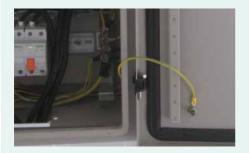
Door of the enclosure is connected physically to the equipotential bonding bar
