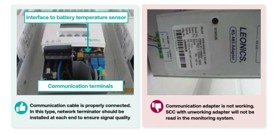
Please refer to the manual for the recommended cable type. Some manufacturer allows only straight ethernet cable type instead of crossover. Using twisted 2 pairs cable for the signal connection may reduce the noise.
