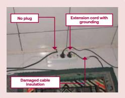
Extension cord should not be placed on the floor. Splash of water might cause very dangerous situation.
