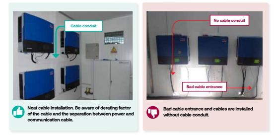
Power cable and communication cable should not be installed close to each other. Installing in the same conduit may introduce noise in the data transmission.
