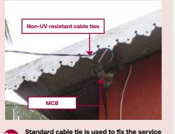
drop cable. MCB should not be installed at the roof.
