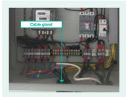
Cable gland is used to prevent animal entering to the panel. It is preferred to have individual gland for each cable.
