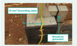
Good grounding of PV mounting structure with proper size and routed nicely. Metallic conduit shoule also be physically grounded.
