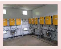
Unfinished floor and untidy cabling. The floor should be added with white ceramic tiles. All the cables should be installed inside cable conduit.
