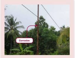
Rusty pole due to poor coating quality. Corrosive pole may lead to reduction of pole strength.
