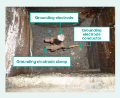
Proper installation of grounding rod. Wellattached grounding electrode and located inside the grounding box.
