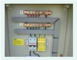
Positive and negative busbars are separated by cable tray.
