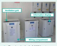
Three Leonics Apollo S-219C inverters are connected in parallel result in 15 kW total output power
