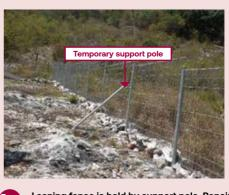
Leaning fence is hold by support pole. Repair the foundation and align the fence.
