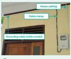
Energy meter box is fixed firmly on the wall with very organized cable installation inside cable conduit and clamp.
