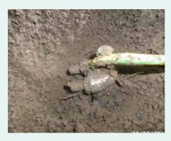
Good quality and corrosion free U-bolt clamp for burrial condition is used. It is preferrable to keep the connection above the ground
