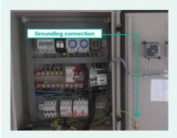
The enclosure including its door is well grounded.
