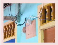
Energy limiter is not installed at the service entrance. Absence of limiter allows unrestrained energy to the owner.
