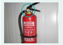
Fire extinghuiser is available on site for emergency case. Needle showing the pressure should be within green area and has to be checked regularly.
