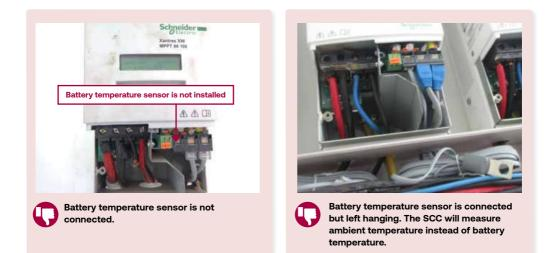
How to install the battery temperature sensor correctly?
