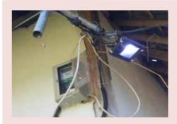
Streetlight is installed in the public building without adequate support and lit during day time.
