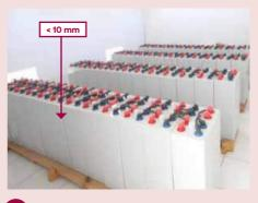
Inadequate distance between battery cells. Minimum distance of 1 cm should be provided.
