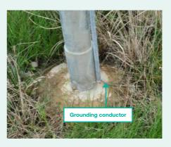
Neutral cable is grounded to maintain the combined PEN conductor at the distribution grid pole.
