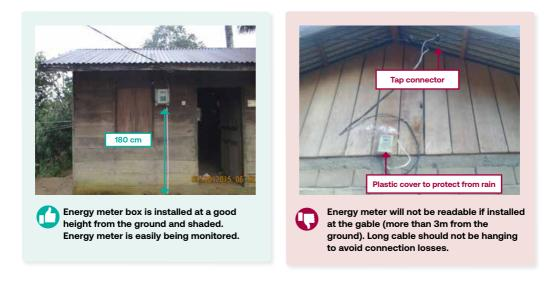
The energy meter box should be accessible both visually and physically by the owner and installed at safe location with minimum 150 cm from the ground.
