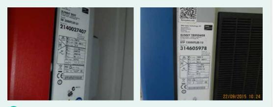
Label attached on the inverter showing the electrical characteristics of the installed grid inverter.
