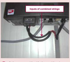
Strings are combined in the combiner box and split equally to be used as input of grid inverter.
