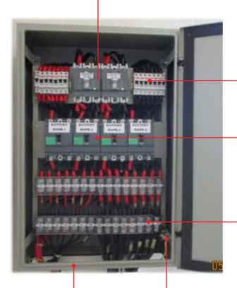
cables from SCC serves additional overcurrent or short circuit protection to the SCC and incoming cable to the panel.
