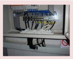
Improper sealant is used at the cable insertion. Cable glands should be used instead.
