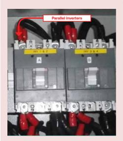
Two inverters are connected in one terminal of three pole MCCB.
