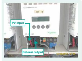
Single cable per terminal and correct cable
