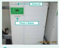
Battery inverters are labelled with ID showing the device type and phase connection
