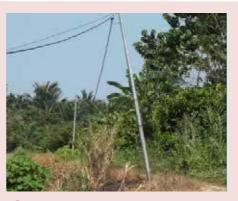
Leaning grid distribution pole due to excessive force at large angle assembly and bad foundation structure.
