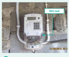
Energy meter with IP 54 is used and sealed. MCB is accessible by the user.
