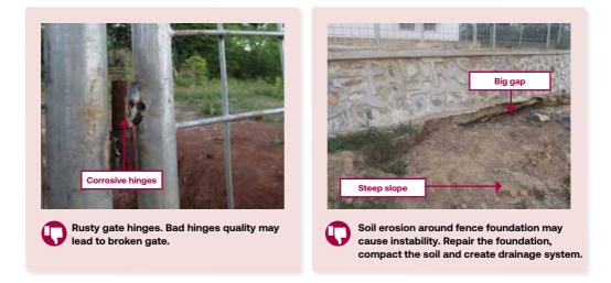
BRC fences have to be coated with zinc (hot-dip galvanized) to avoid rusting especially if installed in the place with high-salinity air.
