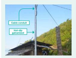
Very good quality pole is used. Pole is made of hot-dip galvanized steel with bigger diameter at the bottom.
