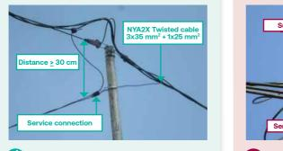
Service connection and main distribution line are installed on different bracket. Adequate distance should be provided.
