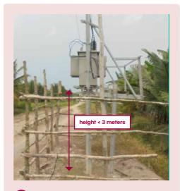
Very low installation of transformer inside inadequate fence. High risk of injury due to electric shock.
