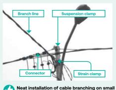
Neat installation of cable branching on smal angle assembly. Proper accessories and connectors are used.
