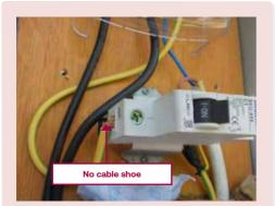
Cable for grounding is used for line connection. The possibility to wrongly connect the cable to the ground is very high.
