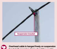
bracket. Suspension clamp should be used to hold neutral conductor of the cable bundle.
