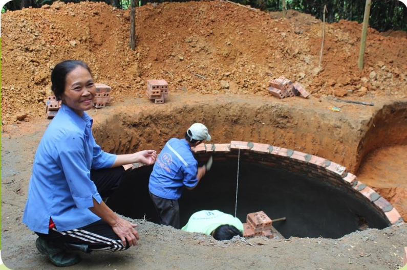
Vietnam: A results-based finance mechanism for biogas enterprises gives the incentive to construct biogas digester like this one.
