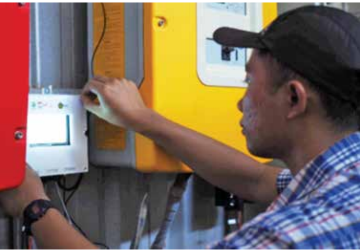
Engineering students of Malang State University were assembling remote monitoring system (left) and installer verifying the correct data on the human machine interface of REMOS hardware on site (right)
