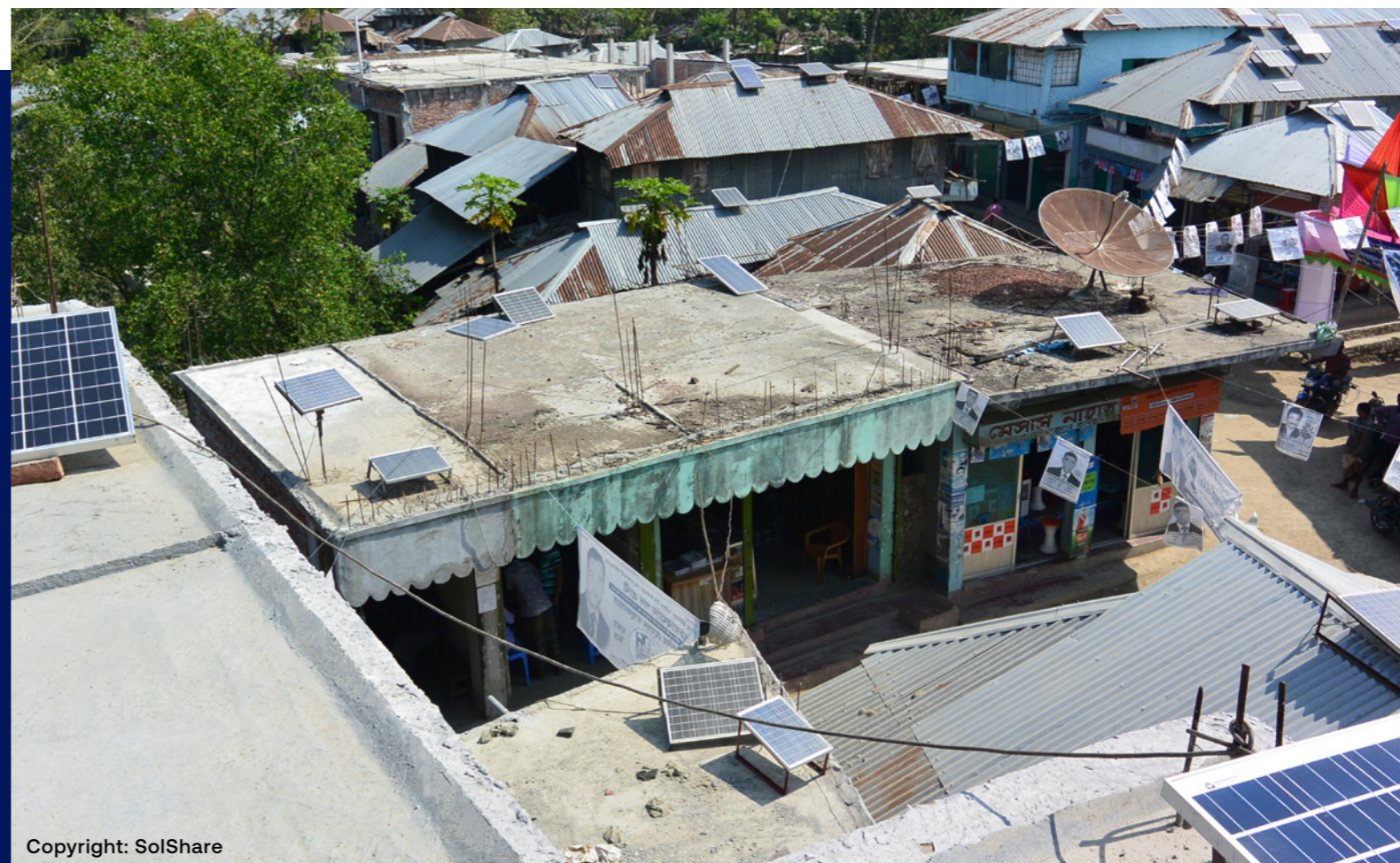
Figure 8. Interconnected solar home systems on Bangladeshi roof tops
