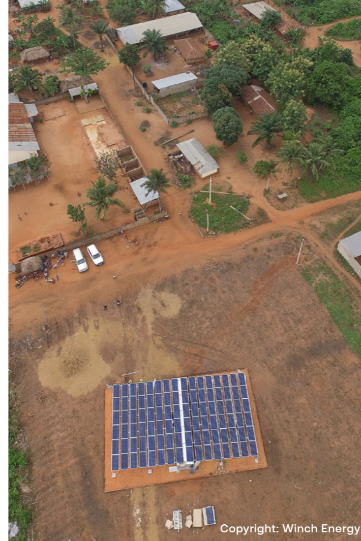
Figure 15. Winch Energy solar mini-grid
