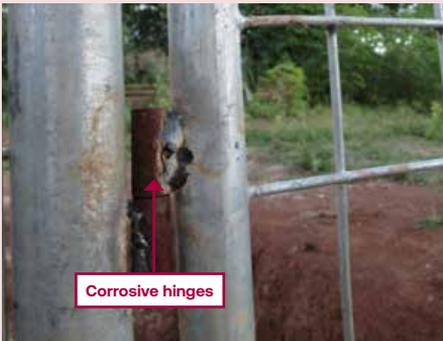
❌ Rusty gate hinges. Bad hinges quality may lead to broken gate.
