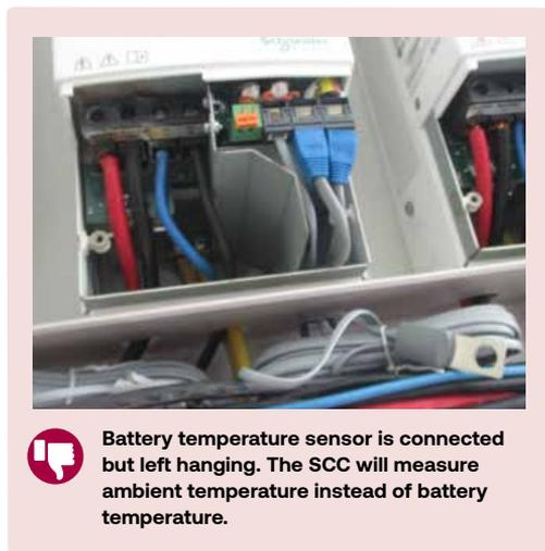
► **How to install the battery temperature sensor correctly?**
