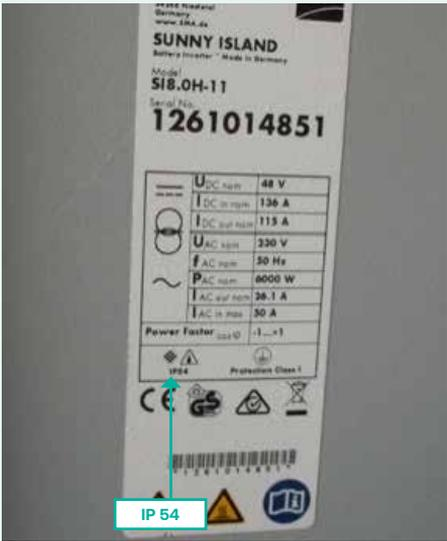
The image shows the technical label of a Sunny Island Battery Inverter, Model 518.0H-11, with serial number 1261014851. The label lists various electrical specifications:
