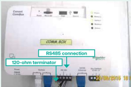
**Pyranometer is connected to Modbus RS485 terminal. Modbus network is terminated by 120 Ω resistor.**
