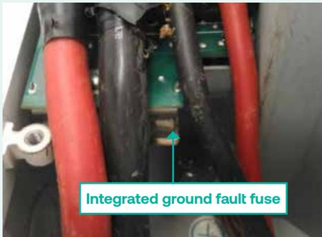
Integrated ground fault fuse
