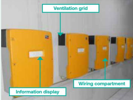
👍 Six SMA Sunny Island 8.0H battery inverters installed in parallel to form 36 kW three-phase AC distribution
