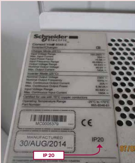
The image shows the technical label of a Schneider Electric Conext XHP 8548 E Inverter. The label lists various electrical specifications:
