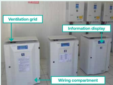
👍 Three Leonics Apollo S-219C inverters are connected in parallel result in 15 kW total output power
