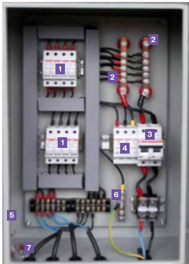
All components in the combiner box is operating in DC voltage that may reach up to 1,000 VDC, depending on the grid configuration. An AC-coupling system with grid inverter typically has higher input voltage of up to 1,000 VDC, while a DC-coupling system with solar charge controller is in the range of maximum 150 VDC. It is preferable and safer to have a lower voltage in PV mini-grid, although higher voltage system will reduce the losses in the circuit.
