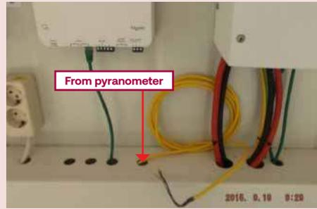
**Pyranometer is installed but not connected to the monitoring device. Avoid installing communication and power cables in the same conduit.**
