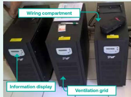
👍 Three Kehua Tech DBX 12-5 kW inverters are installed to provide 15 kW output power to the load
