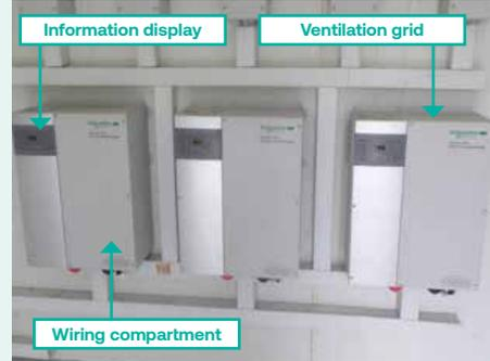
👍 Three Schneider XW 6048 inverters are connected in parallel to achieve 18 kW continuous output power.
