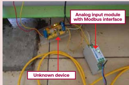
**Messy and unsafe installation of analogue input module from pyranometer.**
