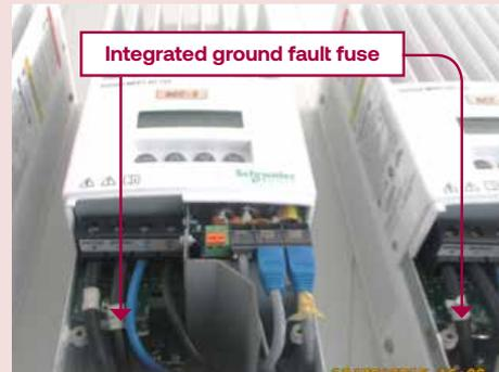
Integrated ground fault fuse
