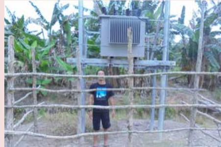
👎 Power transformer is mounted inside easily accessible wooden fence without any warning sign.
