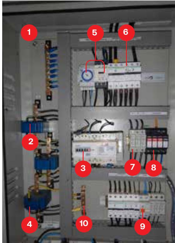
**30 kW AC distribution panel with three-phase configuration**
