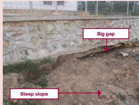
❌ Soil erosion around fence foundation may cause instability. Repair the foundation, compact the soil and create drainage system.
