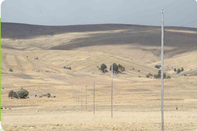
Bolivia: Due to grid densification like here in the department of La Paz, over 270,000 persons gained access to electricity in Bolivia
