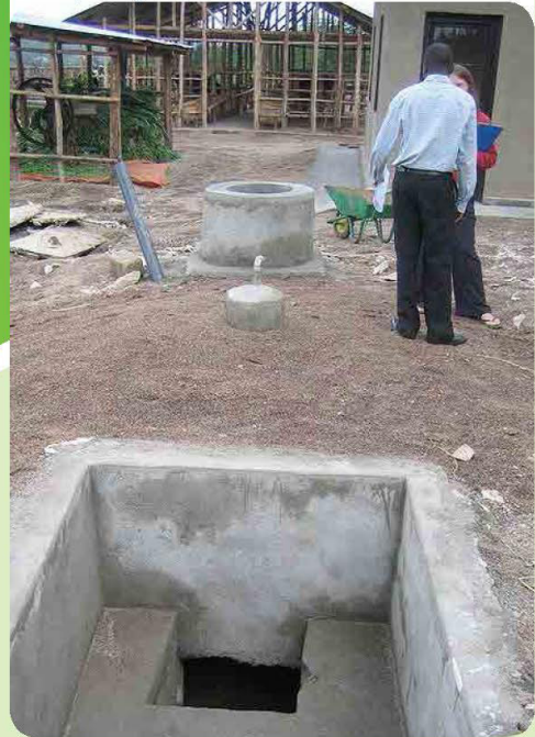
Rwanda: Preparations for the installation of a biogas digester
