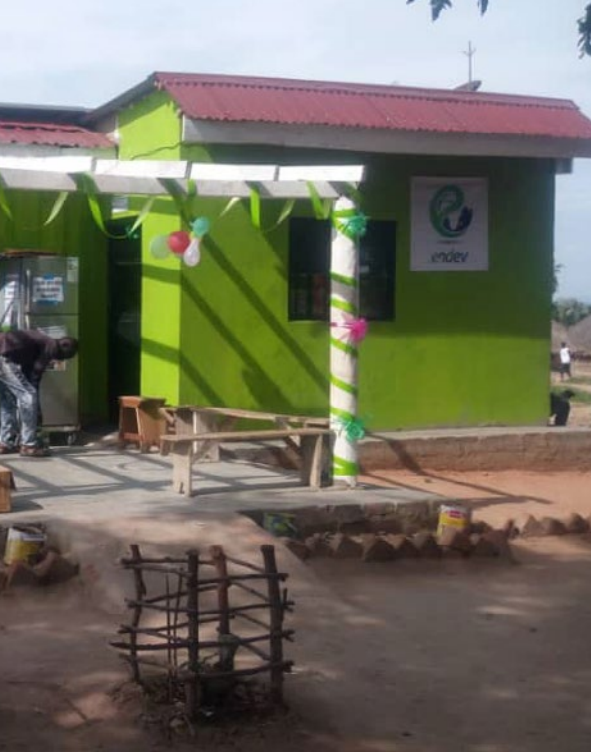
Energy Kiosk in Rhino Camp Refugee Settlement
