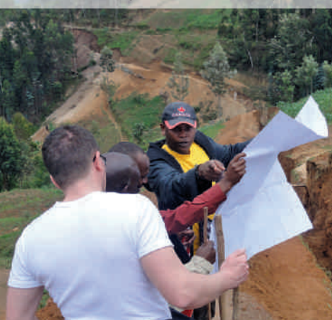
Ruanda: EnDev consultant and project developers discuss at the building site of Mazimeru Micro Hydro Plant.
